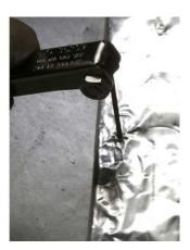
Fig. 10, 11: Find the set screws under the foil insulation and push through with an allen wrench.
